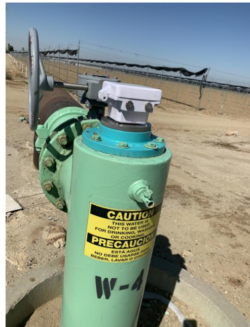
Meter Replacement on Turnout W-4
