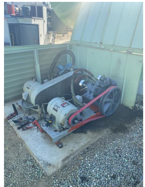
Compressor Pump Repair (N55-P1)
