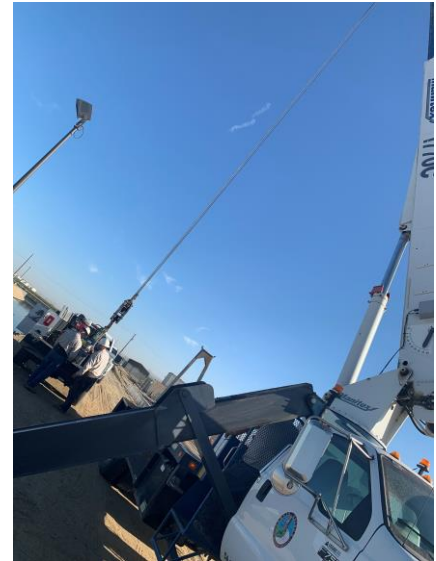
Replacing Gear Box for Check Gate (Tejon Spreading Works)
