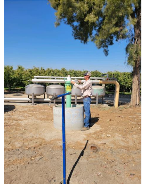
Replacing Meter at Turnout C-112
