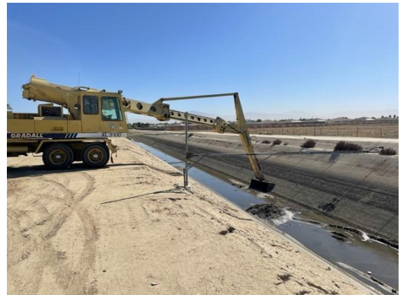
Cleaning of Intake Canal – Winter Maintenance
