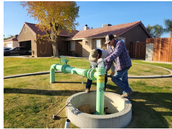
Valve Replacement (E-55)
