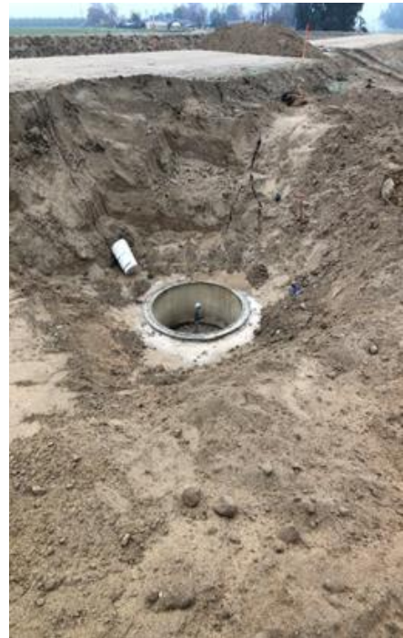
Construction at Forrest Frick Eastside Canal Intertie
