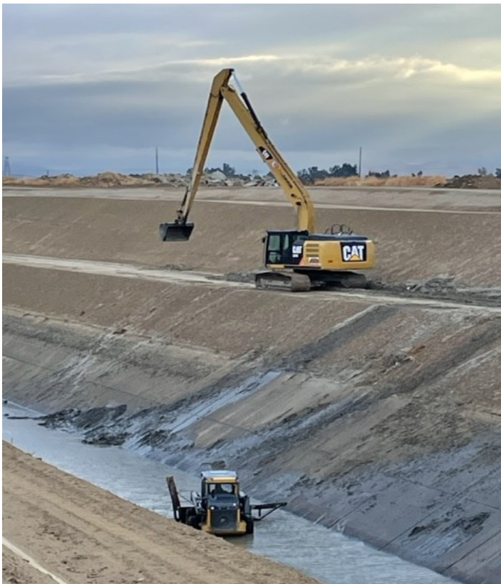
Cleaning of Intake Canal for Winter Maintenance (North Side)
