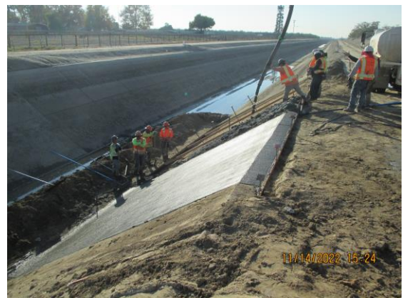
Concrete Liner Repair (Intake Canal)
