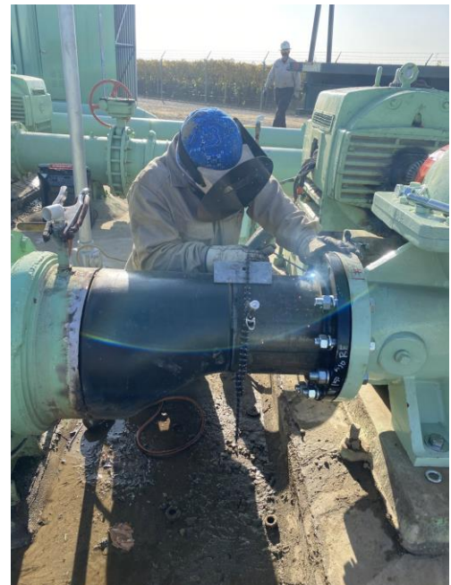
New Pump Installation (N55-P2)
