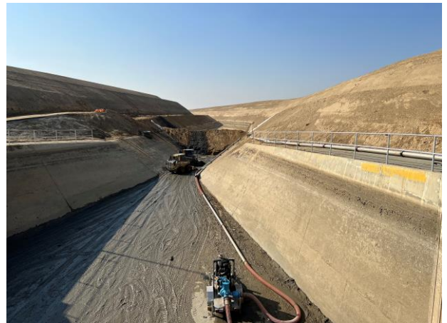
Drained and Cleaned Forebay (FFPP)
