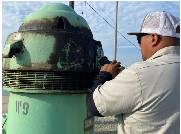
Removing Pump for Repairs (N26-P1)
