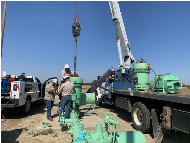
Replacing Failed Motor (Sycamore Well 31)
