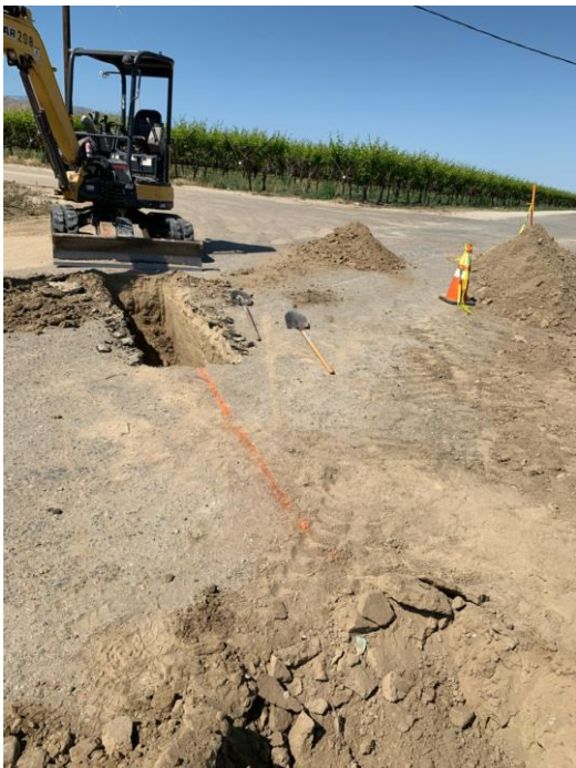
On Site for Underground Service Alert Dig (Lateral S73)
