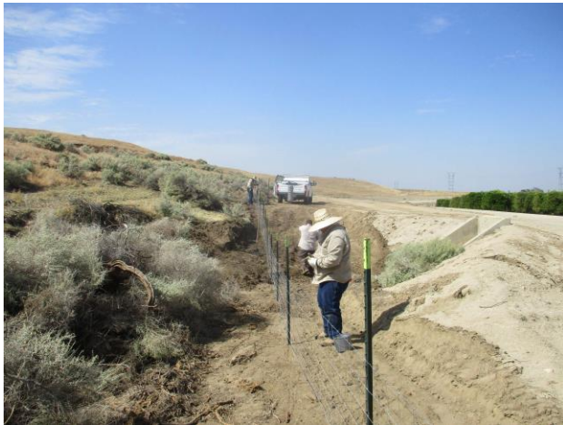
Repairing Fence (South Canal)
