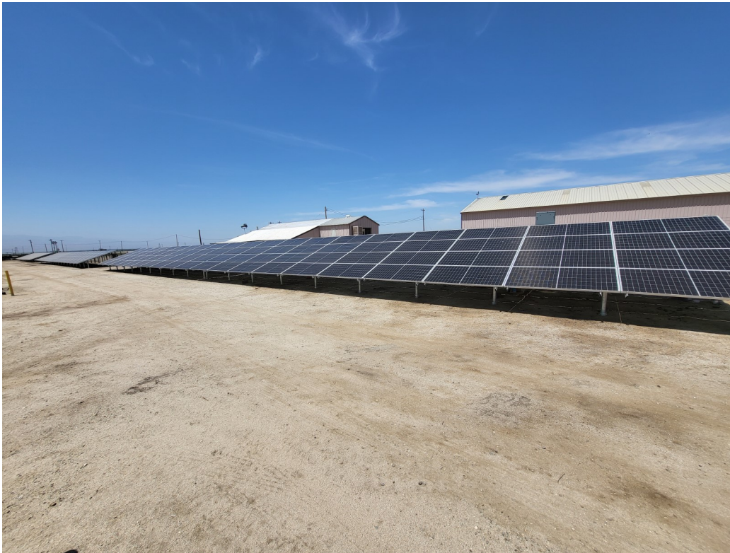
District Headquarters Solar Construction Nearing Completion
