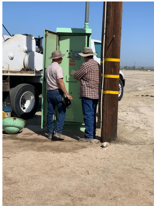
Preparing for Well Startup (Tejon Well 77)
