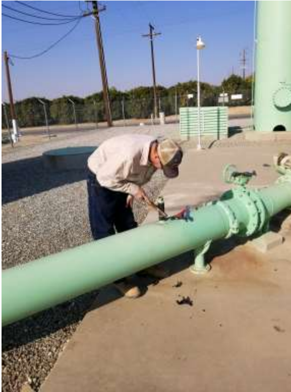
Replacing Ball Valve (N55-P6)
