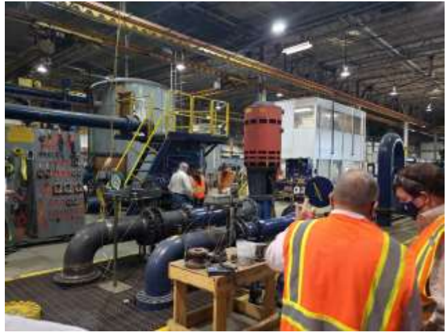
Witnessing 20 CFS Testing (Ruhrpumpen Facility)
