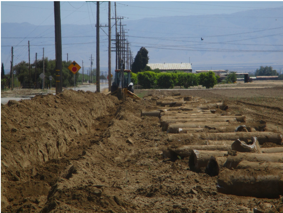
Existing Irrigation Pipeline Removal (Sunset Groundwater Recharge Facility)
