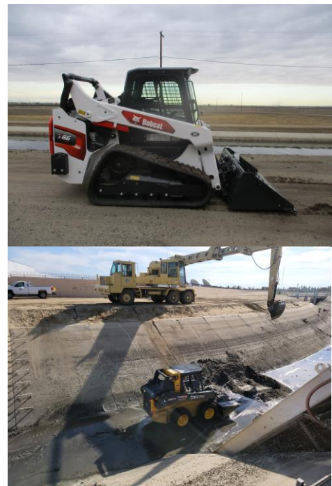
New 2022 Bobcat (Top) & Sediment removal of the Intake Canal (Bottom)
