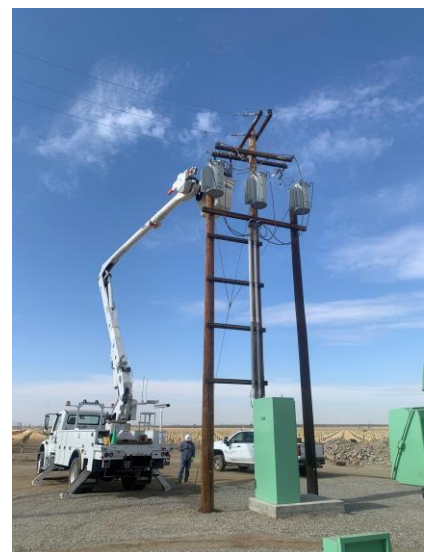
Transformer Replacement at Sycamore Well #38
