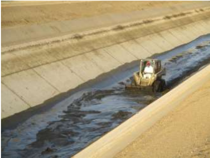
Removing Sediment (North Canal)
