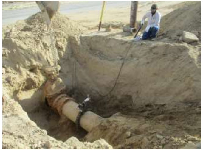
Replacing 18" Isolation Valve (Lateral S73-D)
