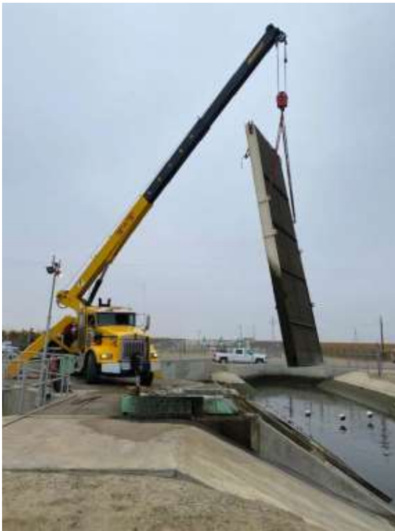
Removing Traveling Water Screens for Repairs (S38-P1)
