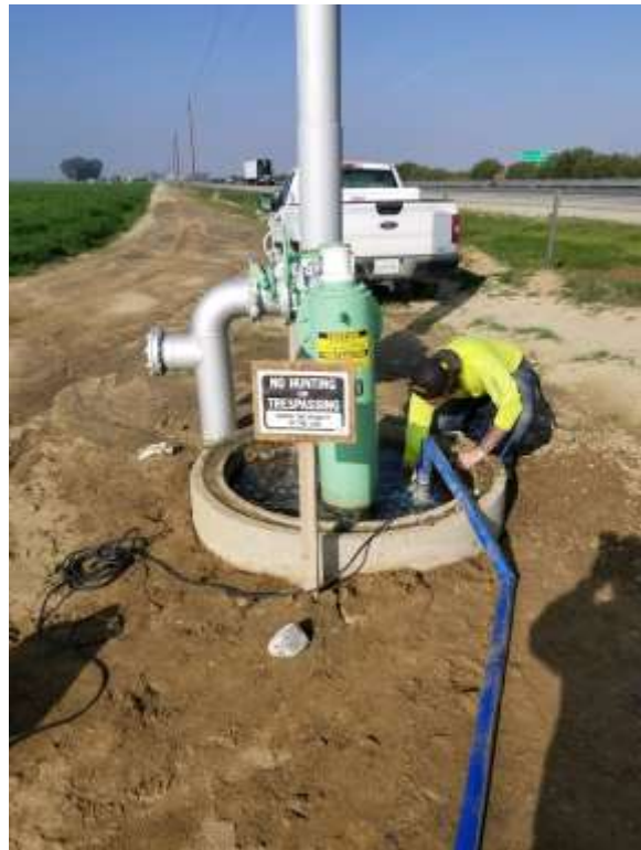
Preparing for Isolation Valve Install (M-10)
