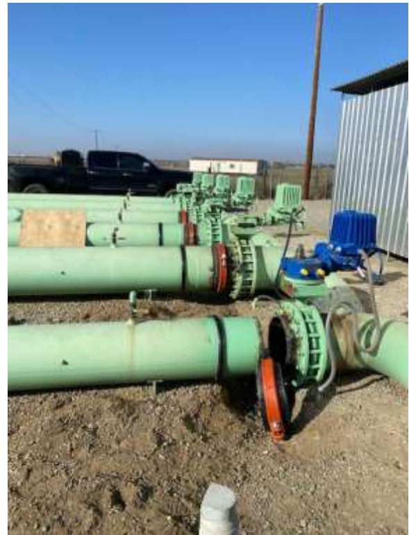
Installing Victaulic Couplers (N55-P1)
