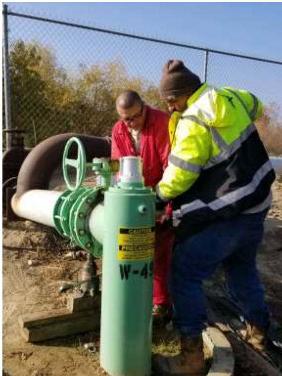
Replacing Valve (W-49)
