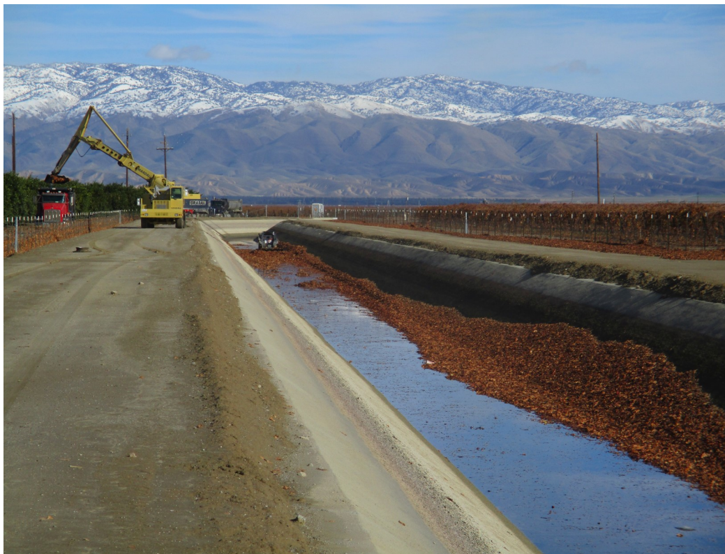
Removing Sediment and Excess Leaves from Canal Prism (South Canal Winter Maintenance Dewatering)
