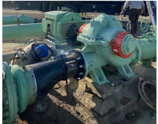
New Reducers and Pipe Joints
