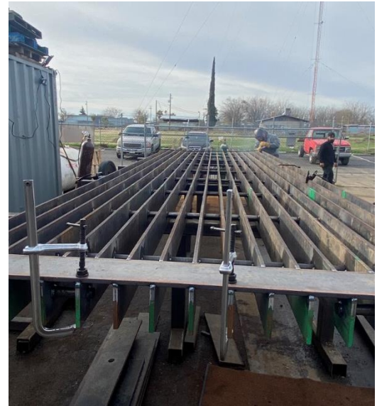
FFPP Trash Rack Fabrication
