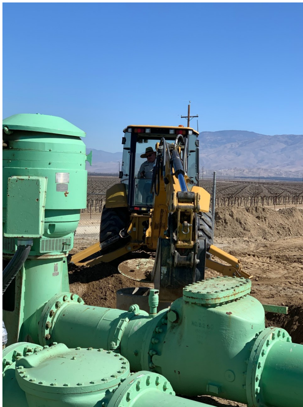
Drainback Valve Replacement (Canalside S73-P1 Pump Plant)
