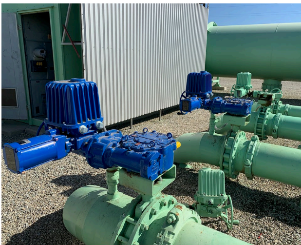
Limitorque Bypass Valves Replaced (N8-P1)
