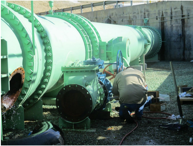
Replacing Bypass Valve (FFPP Unit #3)
