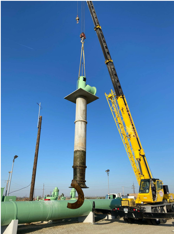
Removal of Failed 50 CFS Unit (Balancing Reservoir Unit #3)
