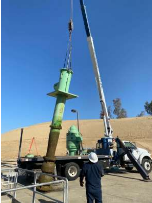
Pump Removal for Repairs (FFPP Unit #7)
