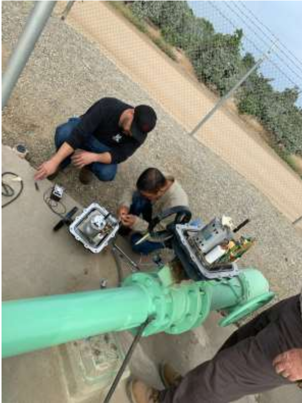
Replacing Bypass Valve Actuator (Pumping Plant N1-P8)
