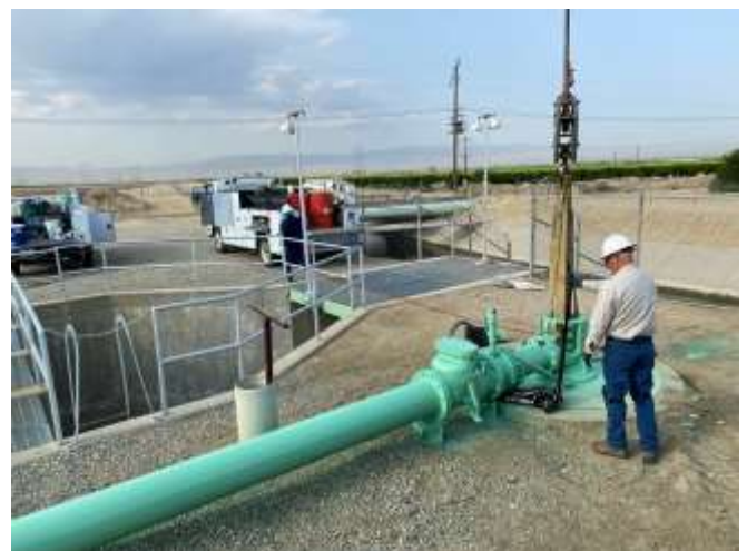
Pump and Motor Replacement (Pumping Plant N8-P1 Unit #5)
