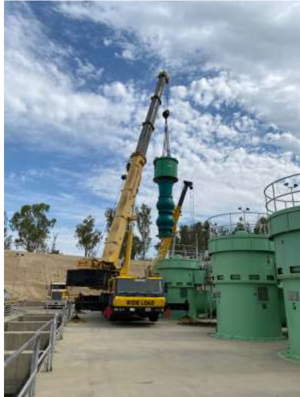
Pump and Motor Installation After Repairs (FFPP Unit #3)
