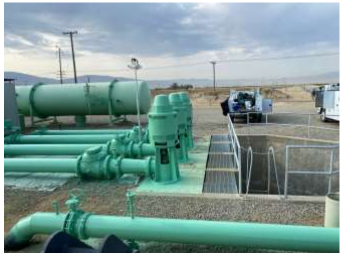
Painting Facilities (Pumping Plant N8-P1)
