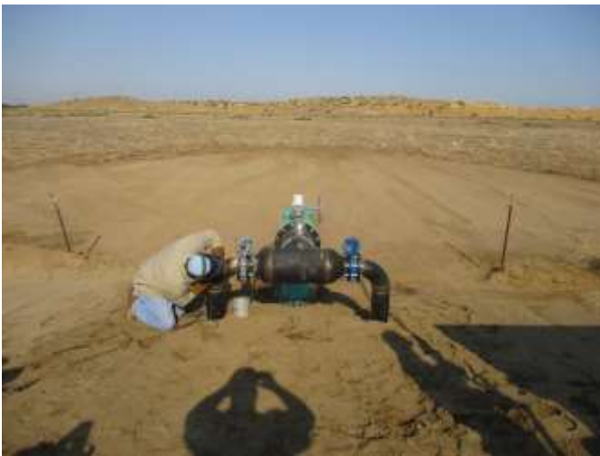
Installing New Turnout for Spreading Operations (Caliente 10-acre Land)
