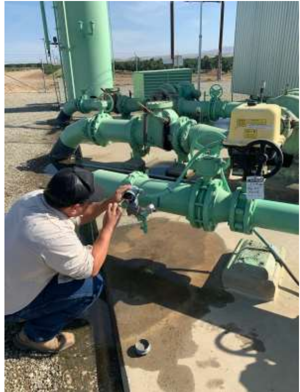
Replacing Bypass Valve Transducer (Pumping Plant N1-P8)
