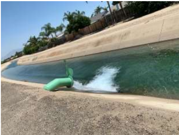
Monitoring Intake Canal Pump-Ins (KD-AE2 into Intake Canal)
