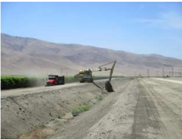
Clearing Out Sycamore Channel Adjacent to South Canal
