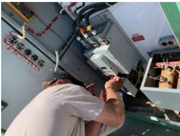
Troubleshooting Well N18 for Startup (North Canal Balancing Reservoir)
