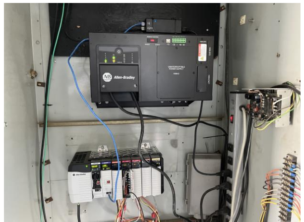
Installation of Batter Backup (Lateral 38)
