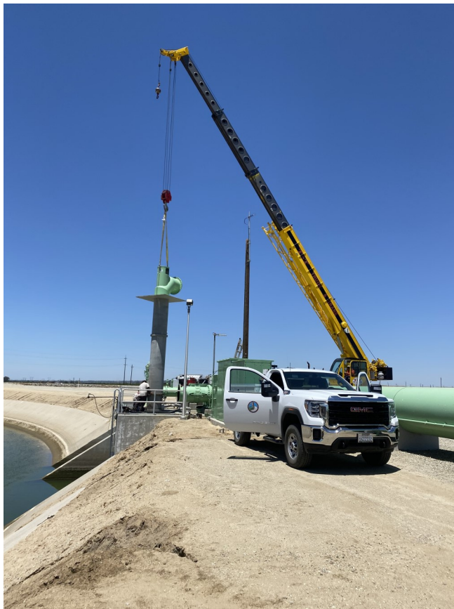
Pump Removal for Repairs (Balancing Reservoir)
