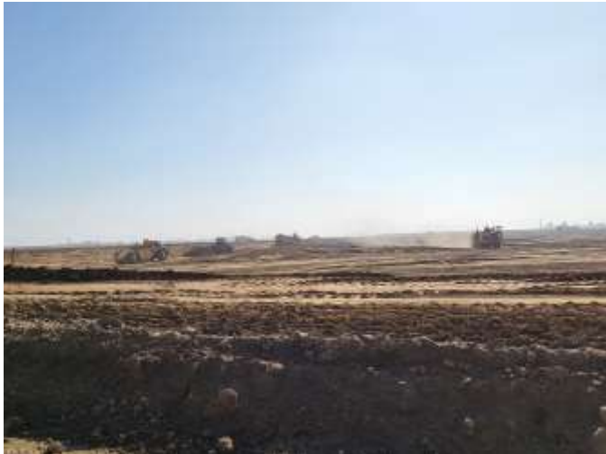
Earthwork Continues (Sunset Spreading Works)
