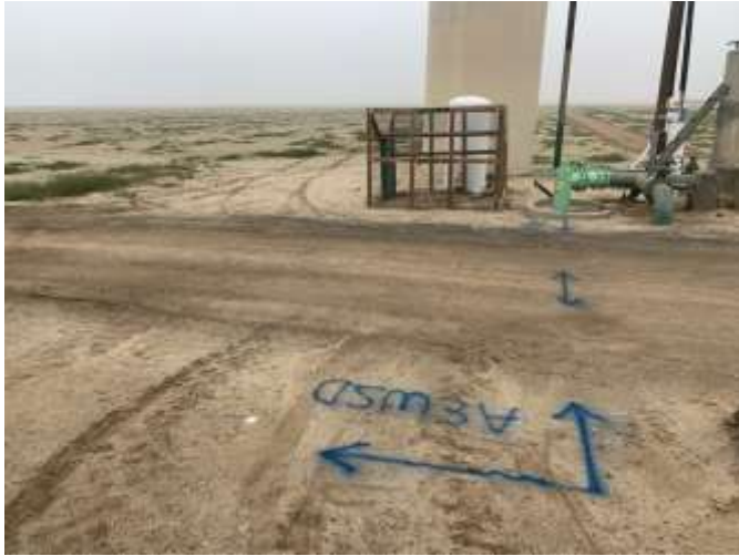
Marking Underground Service Alert Pipelines (W-23)
