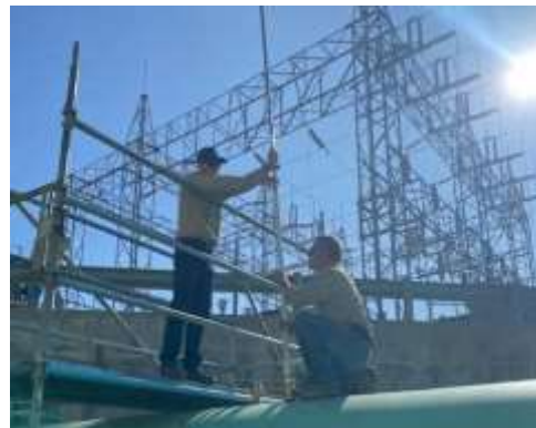
Flow Measurement for FFPP Unit #3 Pump Install (New)
