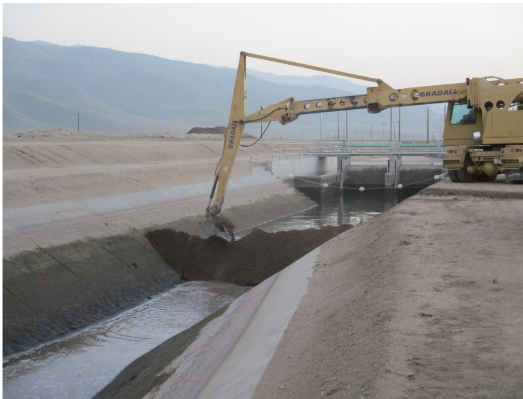
Installing Earth Berm to Isolate North and South Canals for Winter Maintenance Activities (Sycamore Check Structure in Background)
