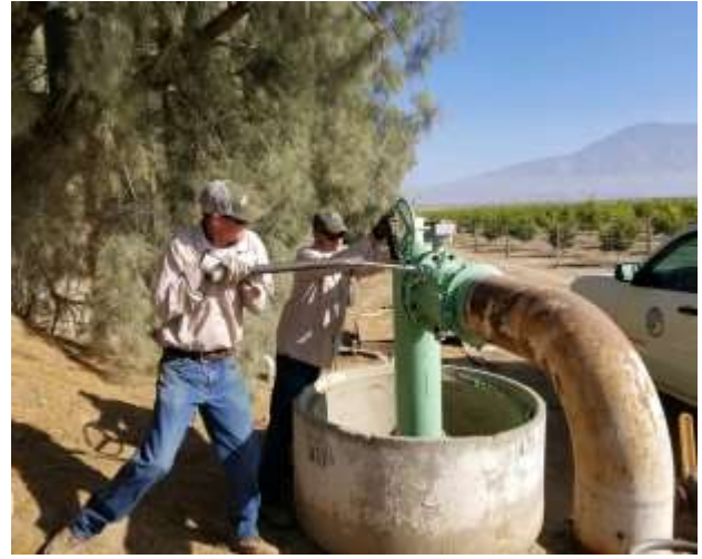
Replacing Turnout Valve (A-71)
