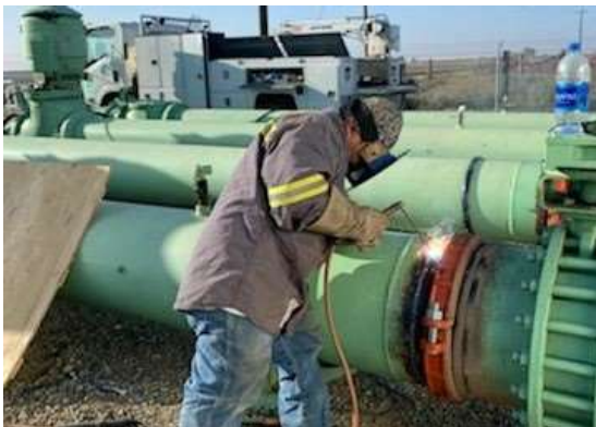
Installing Victaulic Coupler (N55-P1 Unit #4)
