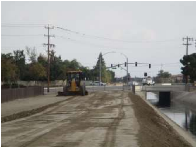
Grading Levees (Intake Canal)
