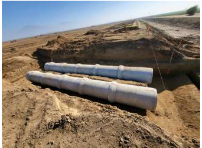
Pipeline Installation for Gravity Pond Diversion (Sunset Spreading Works)
