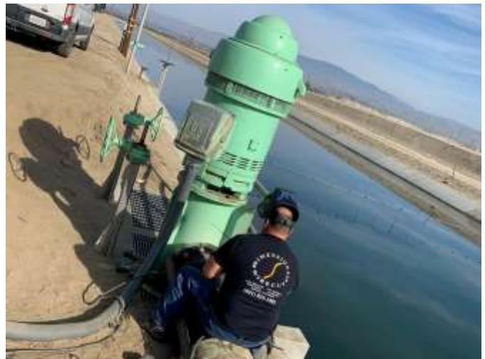
Repairing North Canal Dewatering Discharge Pipeline (Sycamore Check Structure Bypass)
