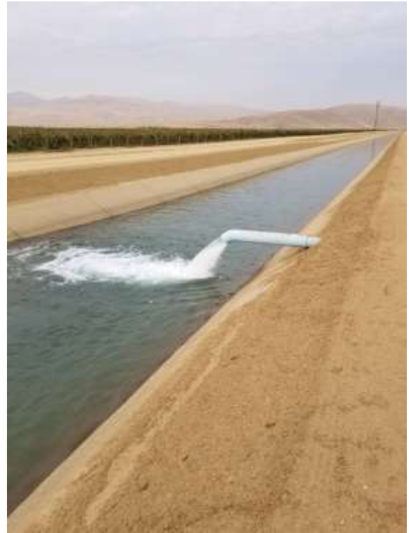
Testing Connection to Wheeler Ridge-Maricopa WSD 850 Canal (Turnout W-63)
