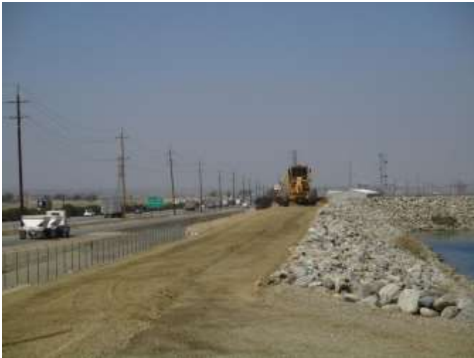
Grading Levees (Spillway)
