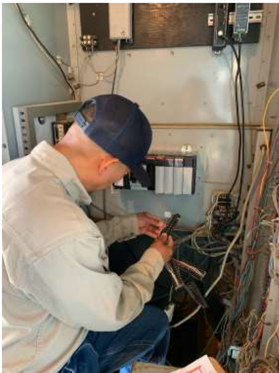
Installing New Level Sensor (Spillway)
