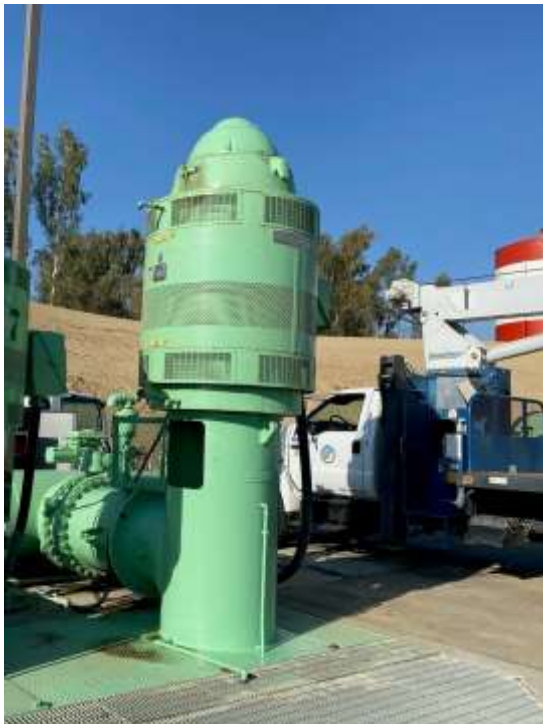
Unit #8 Pump Installed After Repairs (FFPP)
