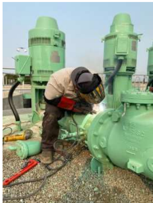
Welding Coupler for Discharge Piping Repair (N8-P1 Unit #4)
