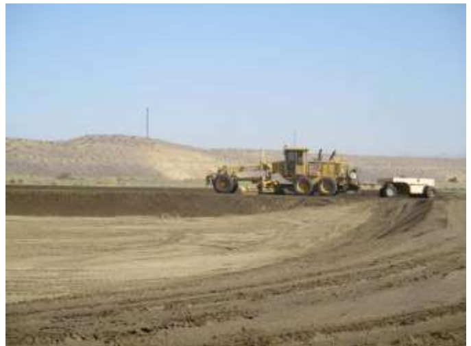
Earthwork Continues at District-Owned 10 Acres Site (Caliente Unit)
