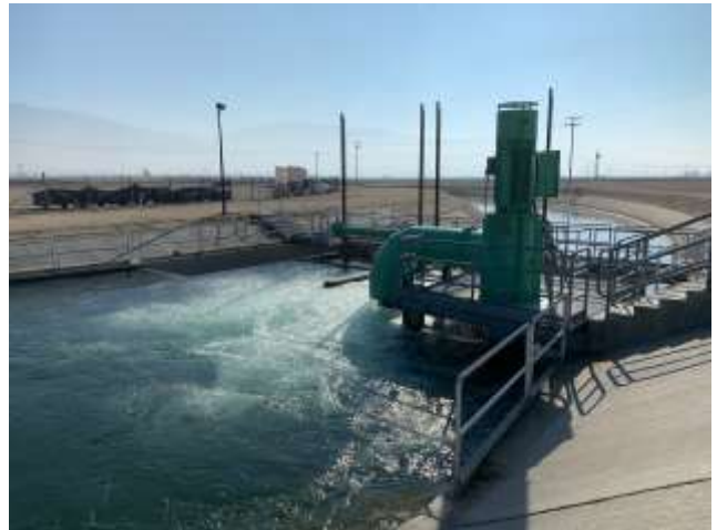
Operating North Canal Pumpback After Troubleshooting
