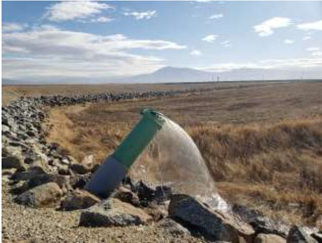
Balancing Reservoir Wells Startup Testing (N15)
