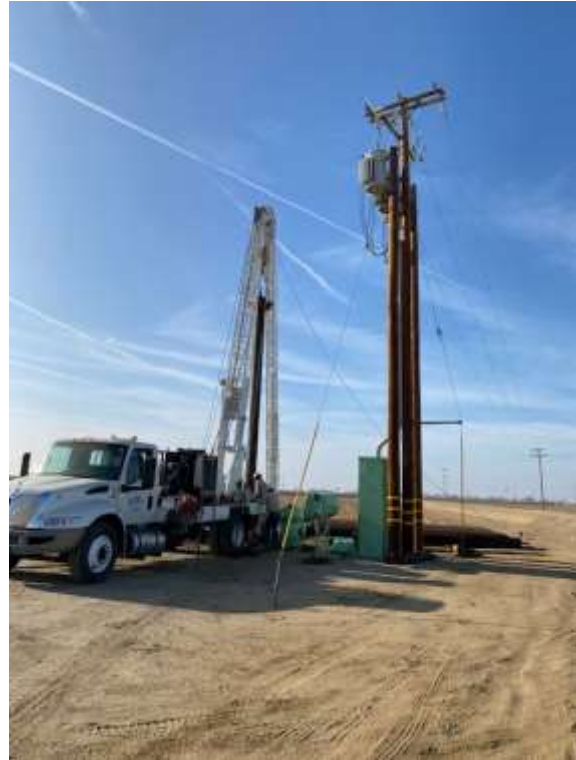
Well Repairs Underway (N11)
