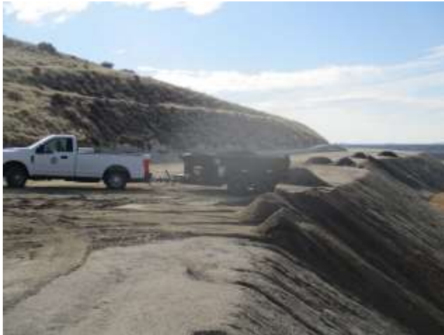
Repairing Washouts (South Canal)
