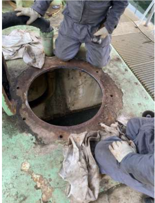
Removing Pumps for Base Plate Modification in Preparation for New Pump Bowls
