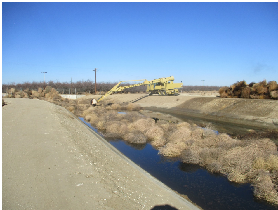
Cleaning Out Canal (Wind Storm Debris)
