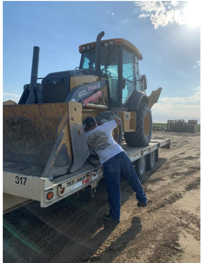
Unloading Backhoe for Pipeline Repair (Lateral S93)
