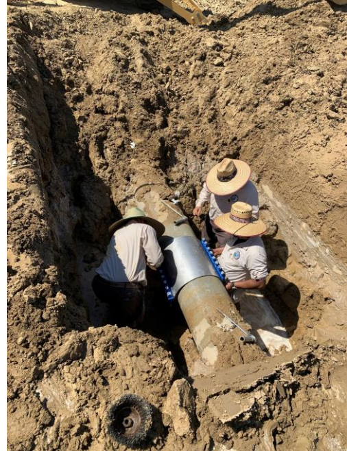
Pipeline Repair at Turnout M-25 (Lateral S93)
