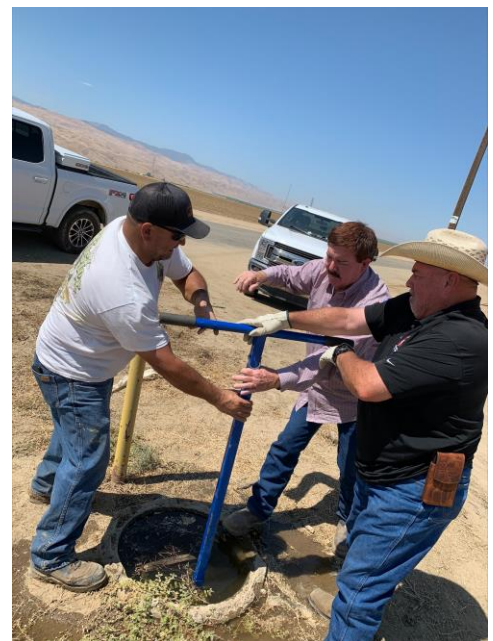
Closing Isolation Valve for Line Repair (Lateral S93)
