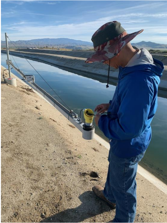
Replacing Water Level Transducer (Sycamore Checkgate)
