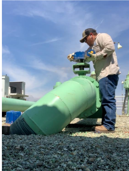
Repairing Limitorque (S38-P1)
