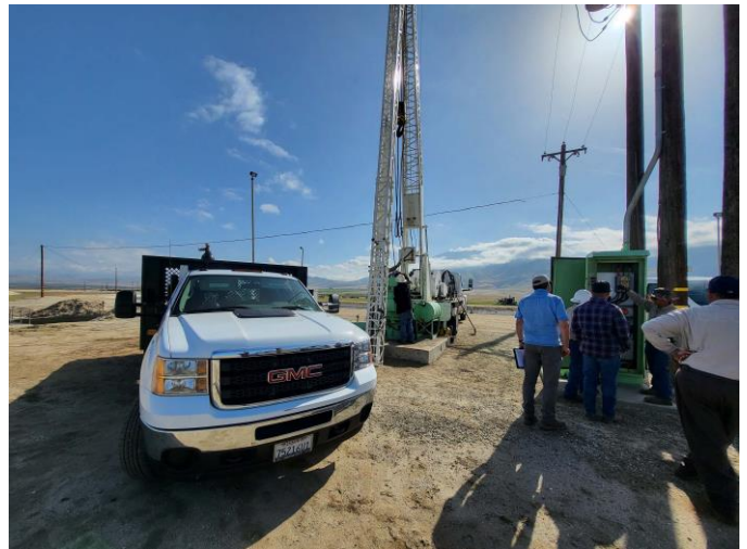
Staff and Consultants Onsite for Well Startup (Sycamore #8)
