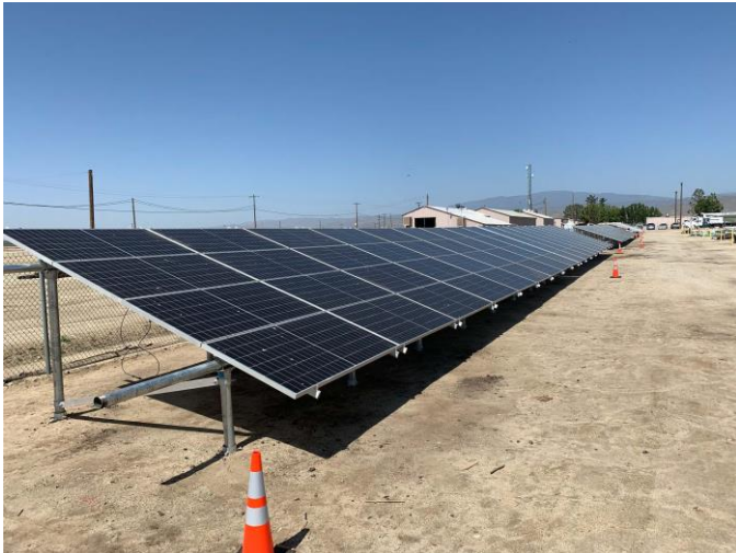
Solar Panel Construction In Progress (Headquarters)
