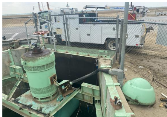
Removing Pump for Repairs (N26-P1)
