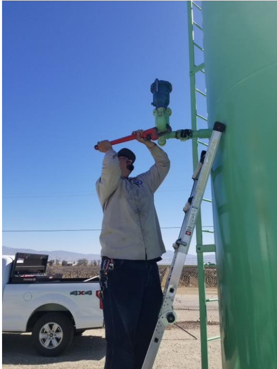
Replacing Air Vent (S93-P2)
