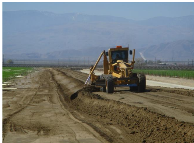
Grading In Preparation for Fence Install (South Canal)
